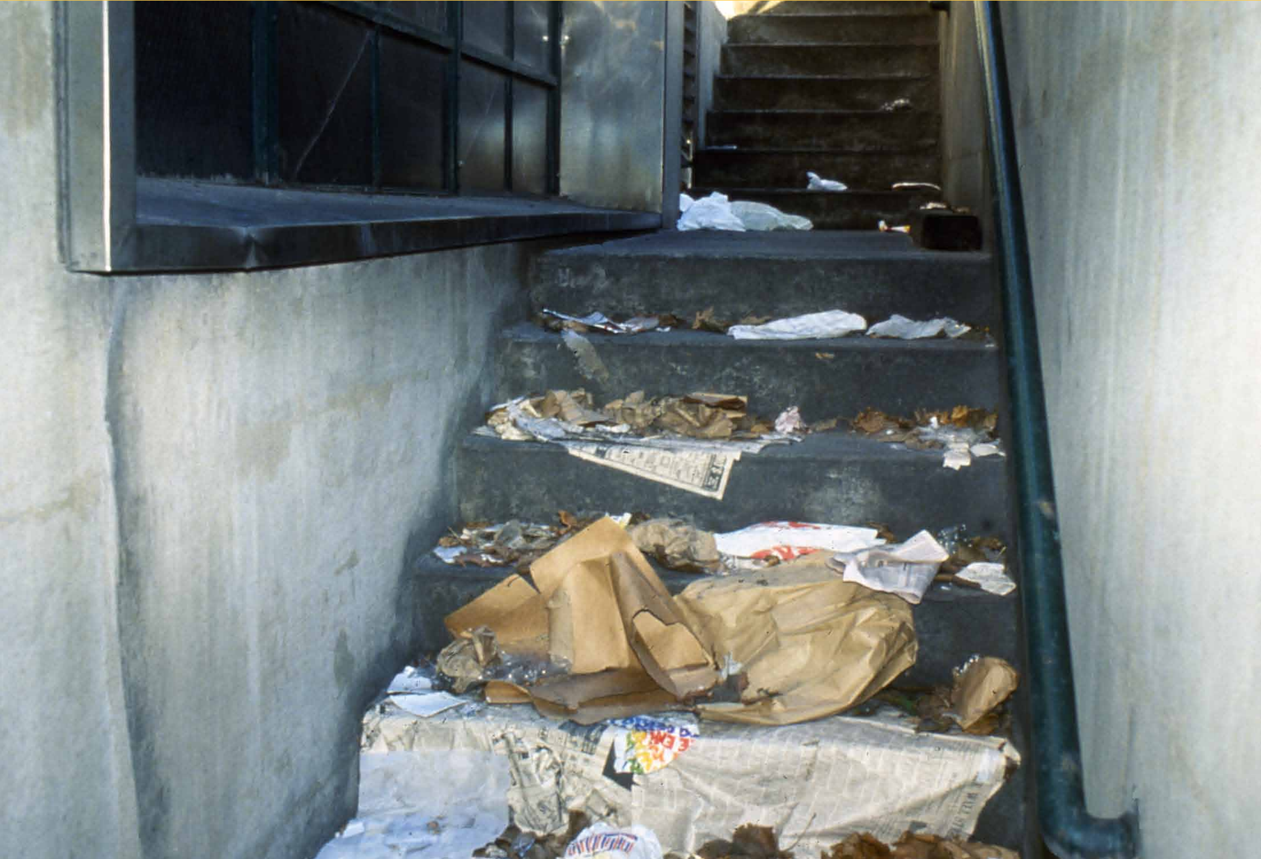
City of Boston Parking Garage Unit 3 was not as well maintained as the Norman B. Leventhal Park. Be glad this photo is not a scratch & sniff!
